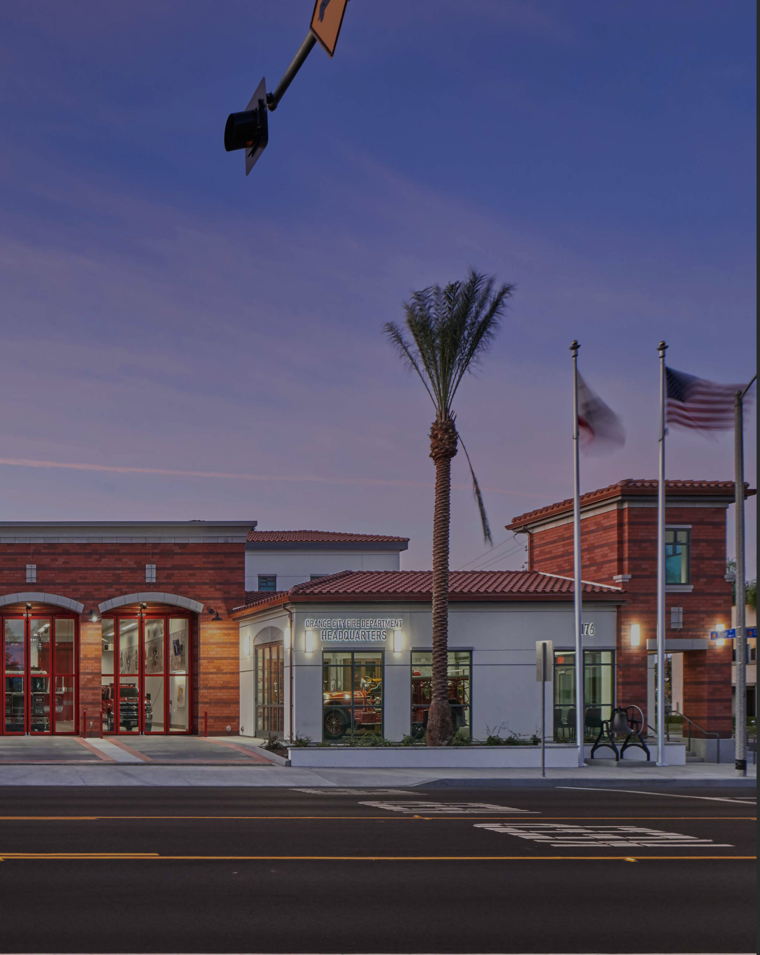
ORANGE CITY FIRE DEPARTMENT HEADQUARTERS & STATION 1
