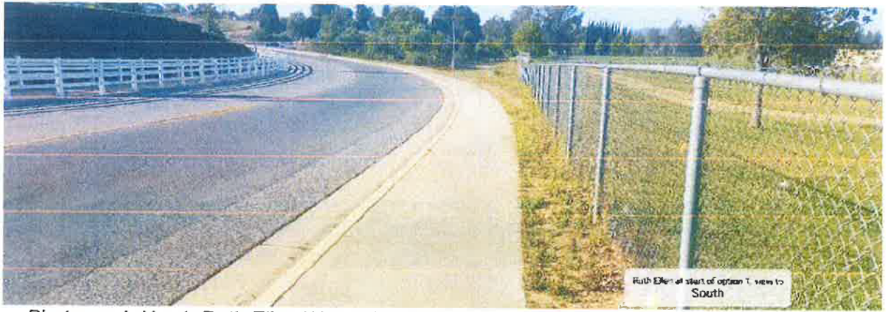
Photograph No. 1: Ruth Ellen Way at beginning of pipeline alignments BH-02, facing south.
