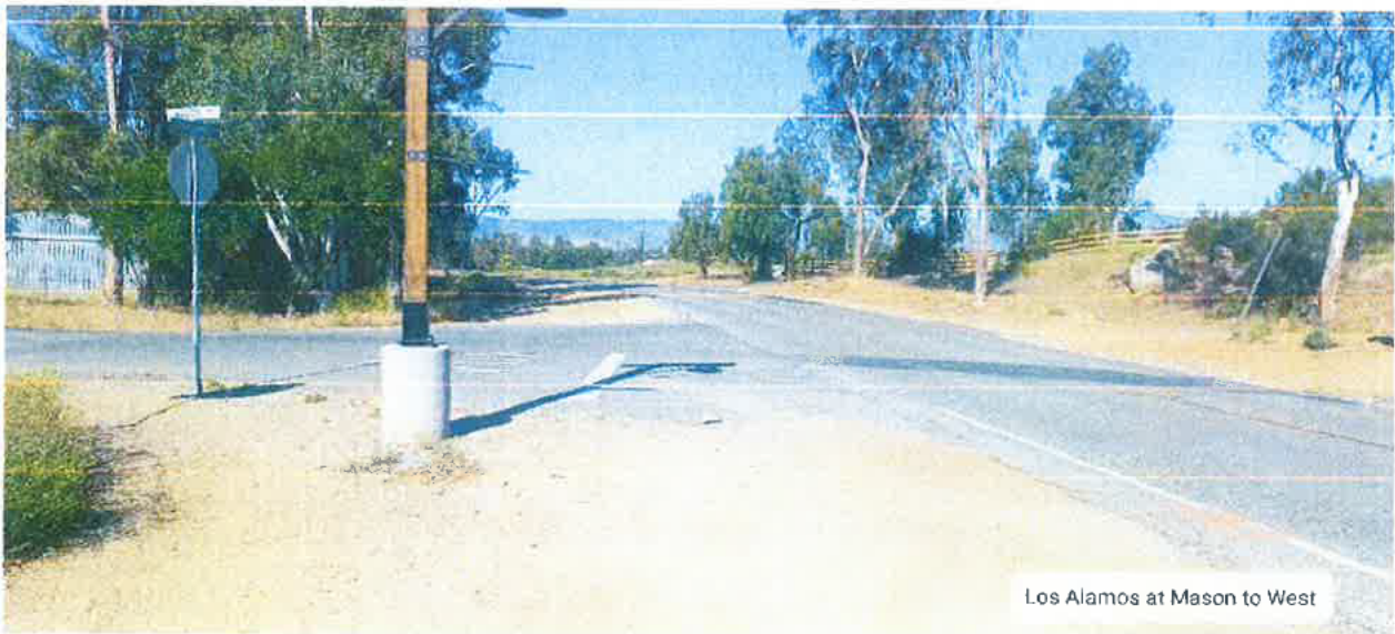
Photograph No. 6: Los Alamos Road at Mason Avenue (BH-12), facing southwest.
