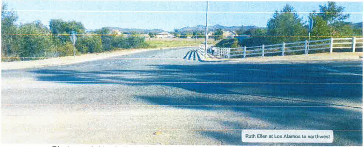
Photograph No. 2: Ruth Ellen Way at Los Alamos Road, facing north.
