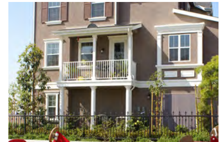
Private open space at upper level
