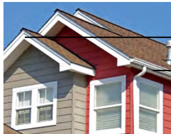
RAKE OVERHANGING EAVE OVERHANGING
