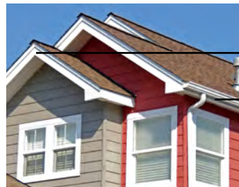
RAKE OVERHANGING EAVE OVERHANGING
