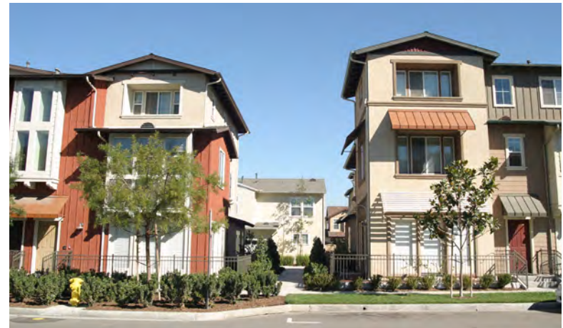
Large residential complex developments shall provide diversity through different architectural styles or colors.
