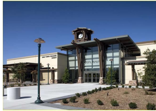
Figure 4.1.6 – Murrieta City Hall
