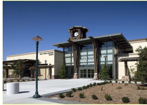
Figure 4.1.6 – Murrieta City Hall
