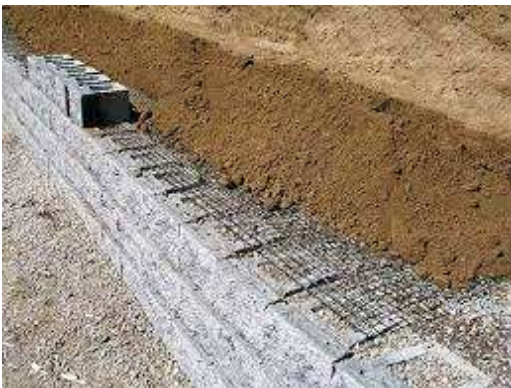
Image 1 - Geogrid Wall Installation
