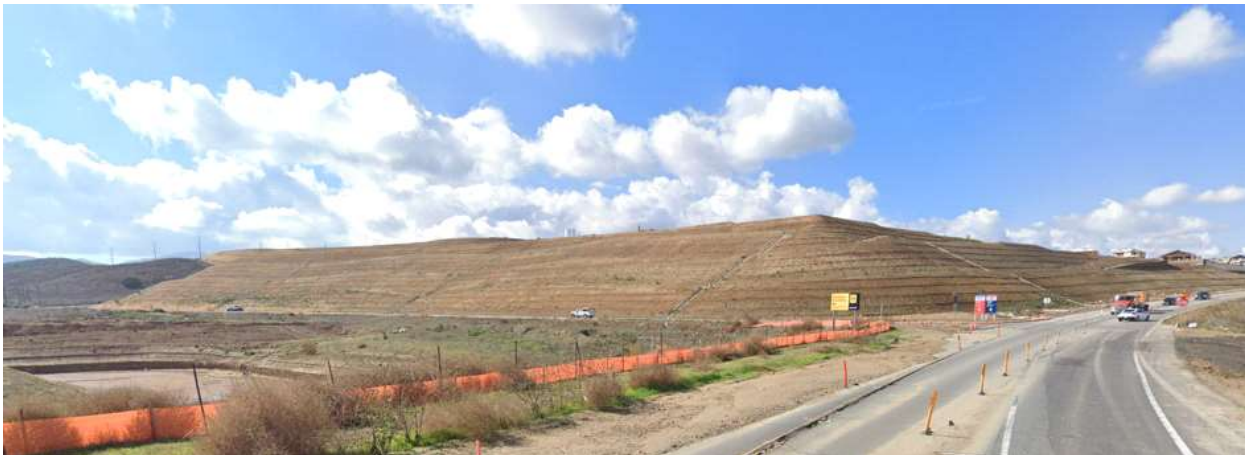
Image 10 - Earlier in the Development of the Project - Example of mass-grading hillsides that don't blend into a hillside with hard edge lines.
