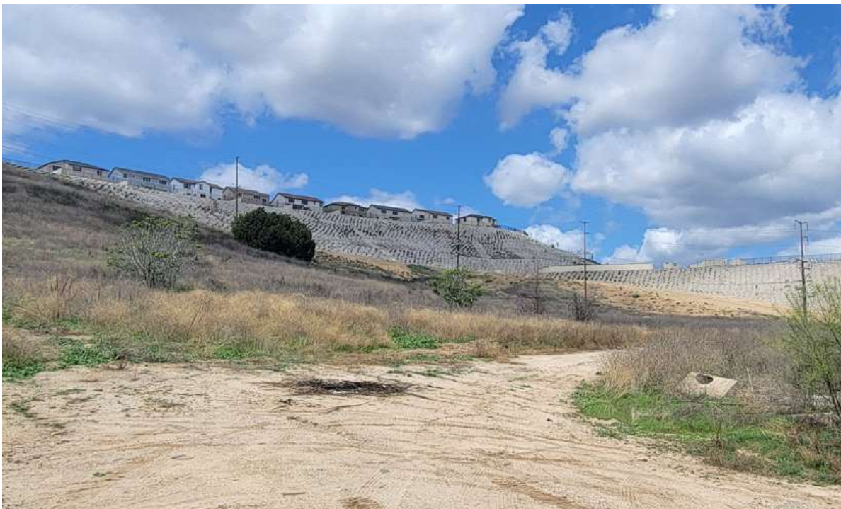
Image 12 - Example of manufactured hillsides that do not blend into a hillside with hard edge lines.
