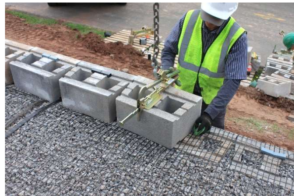
Image 2 - Geogrid Wall Installation
