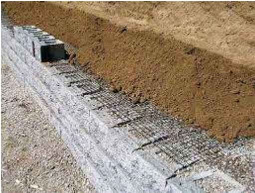
Image 1 - Geogrid Wall Installation
