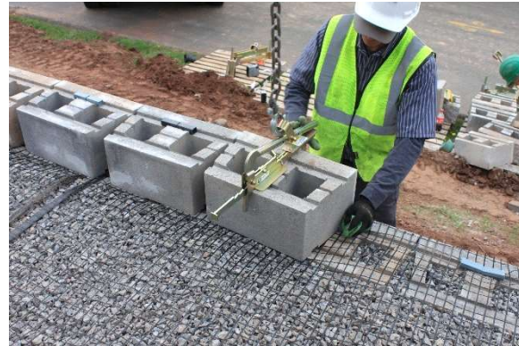
Image 2 - Geogrid Wall Installation
