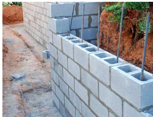
Image 3 - Conventional Retaining Wall Installation
