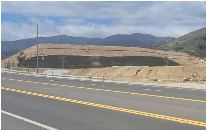
Images 5 and 6 - Examples of Tall Retaining Walls at highly visible locations
