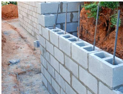
Image 3 - Conventional Retaining Wall Installation
