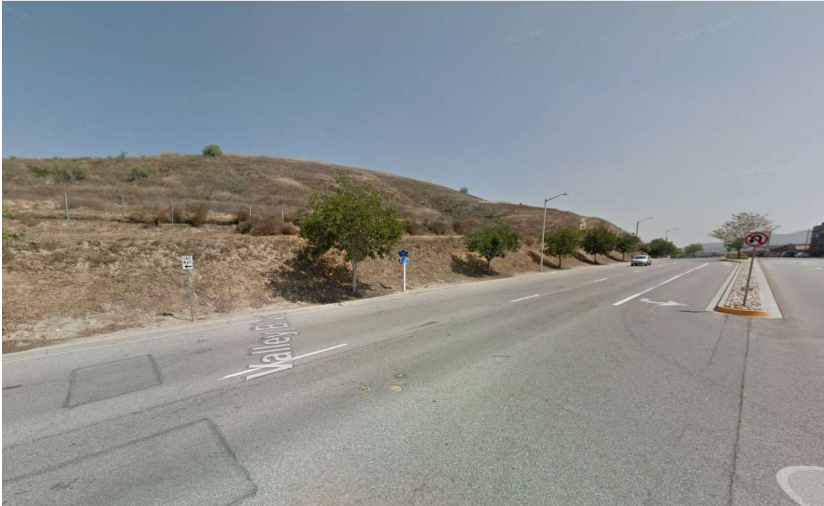
Image 13 - Before - Example of over-excavation/retaining walls that do not blend into a hillside with hard edge lines.
